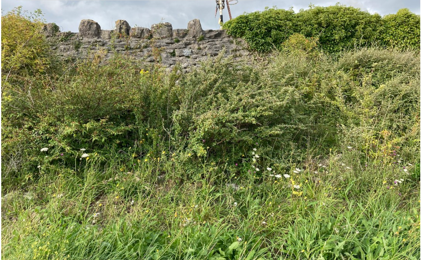
Views summer 2023 before clearance work
