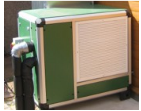
Air Source Heat Pump
